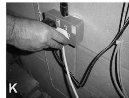
Isolate From Mains Supply
